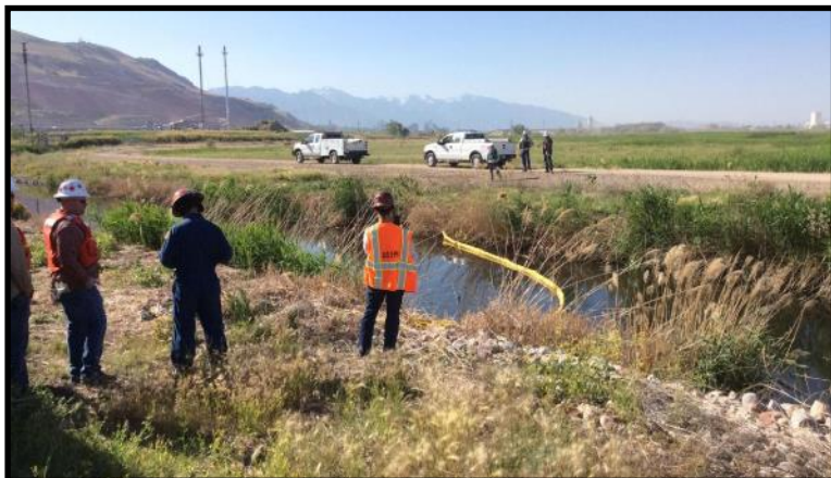
Setting Boom in Oily Water Canal
