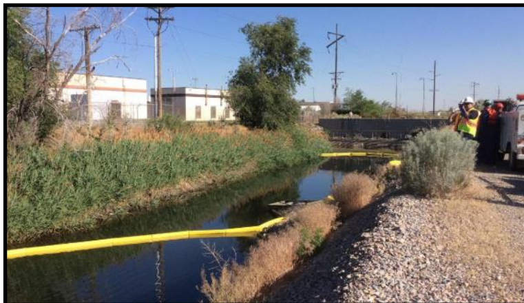
Setting Boom in Oily Water Canal
