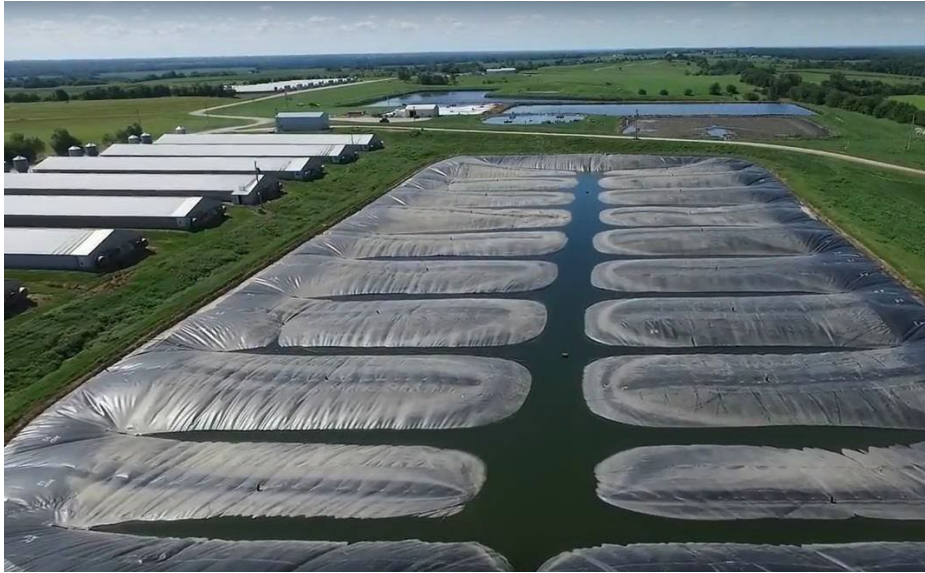
Aerial view of covered manure lagoons. Photo Credit: Roeslein Alternative Energy, LLC
