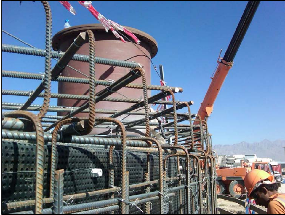
Photograph 2.2-11 Geosynthetic drainage layer (black material with dimples).
