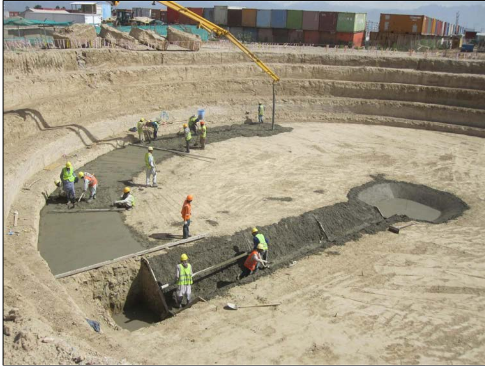
Photograph 2.2-1 Excavation and initial leveling course.
