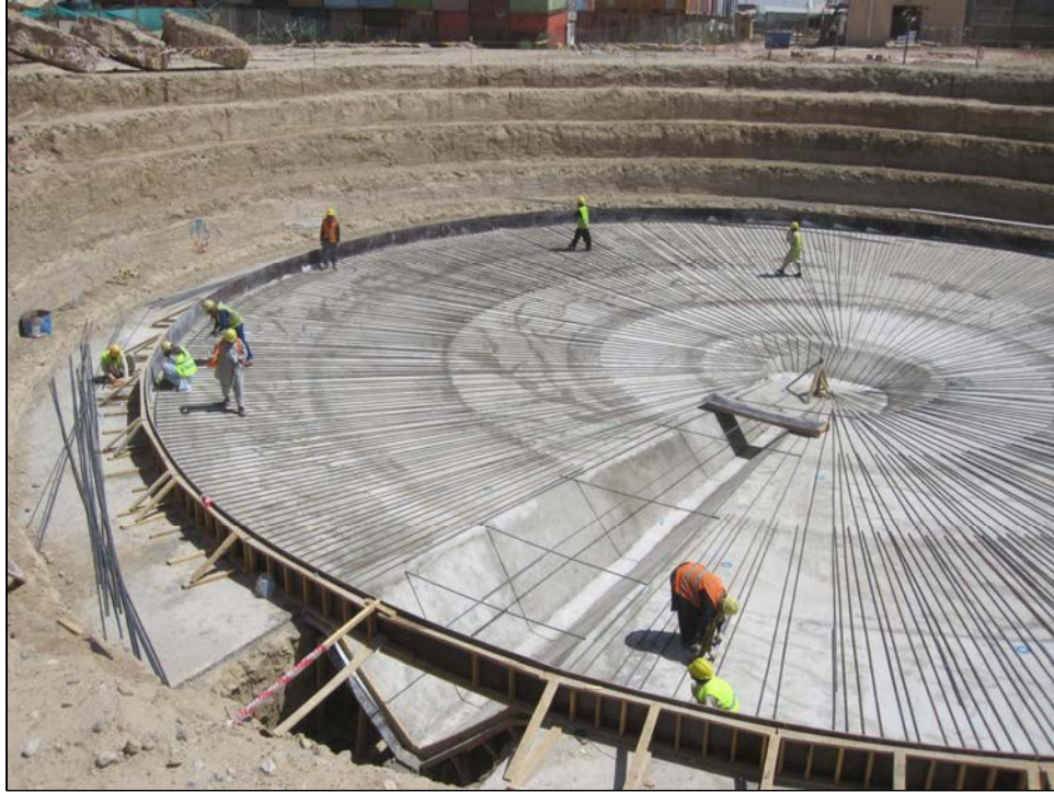
Photograph 2.2-5 Installation of rebar for reinforced concrete foundation slab.
