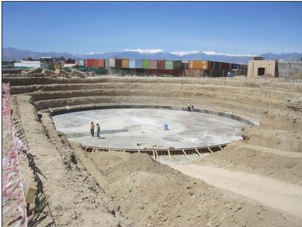
Photograph 2.2-2 Completed leveling course.
