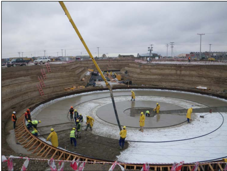
Photograph 2.2-4 Protective grout course.
