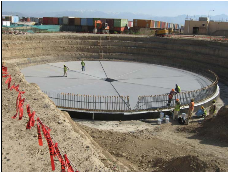
Photograph 2.2-6 Completed foundation slab with radial drainage gutters.
