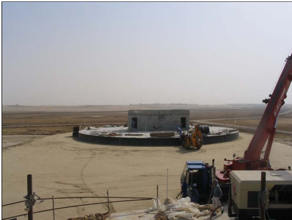
Photograph 2.2-12 Completed underground vertical (cut-and-cover) storage tank.
