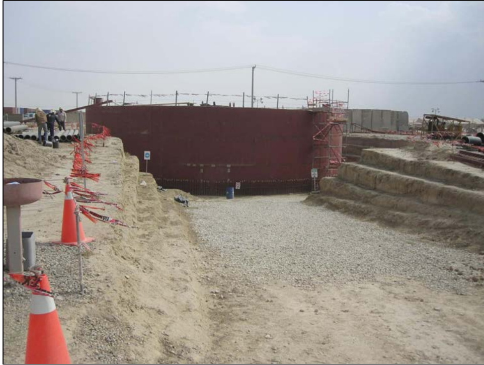
Photograph 2.2-9 Completed welded steel tank.
