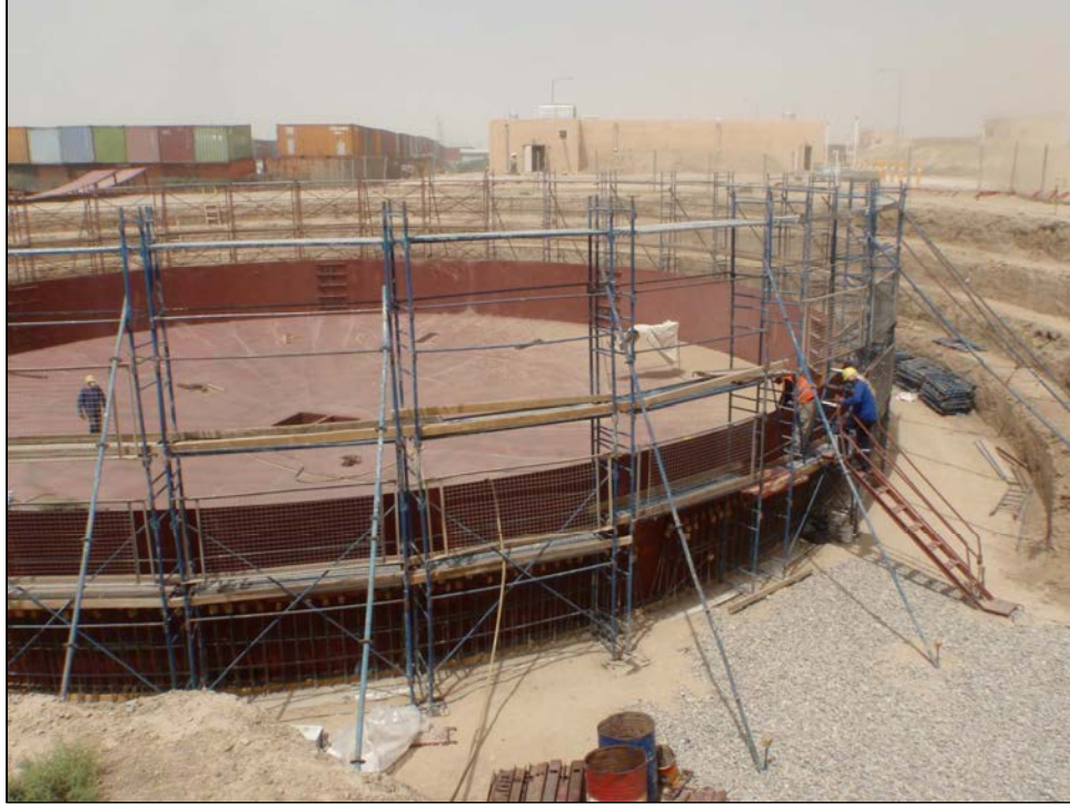
Photograph 2.2-7 Welded steel tank bottom and first shell course.
