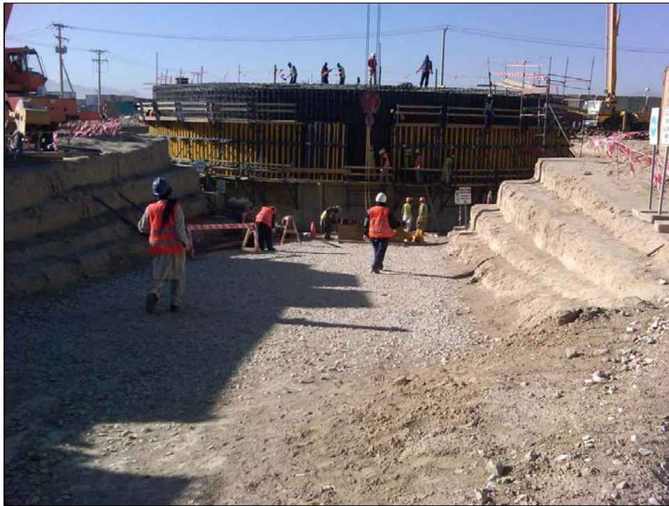
Photograph 2.2-10 Initial formwork and rebar placement for concrete secondary containment.
