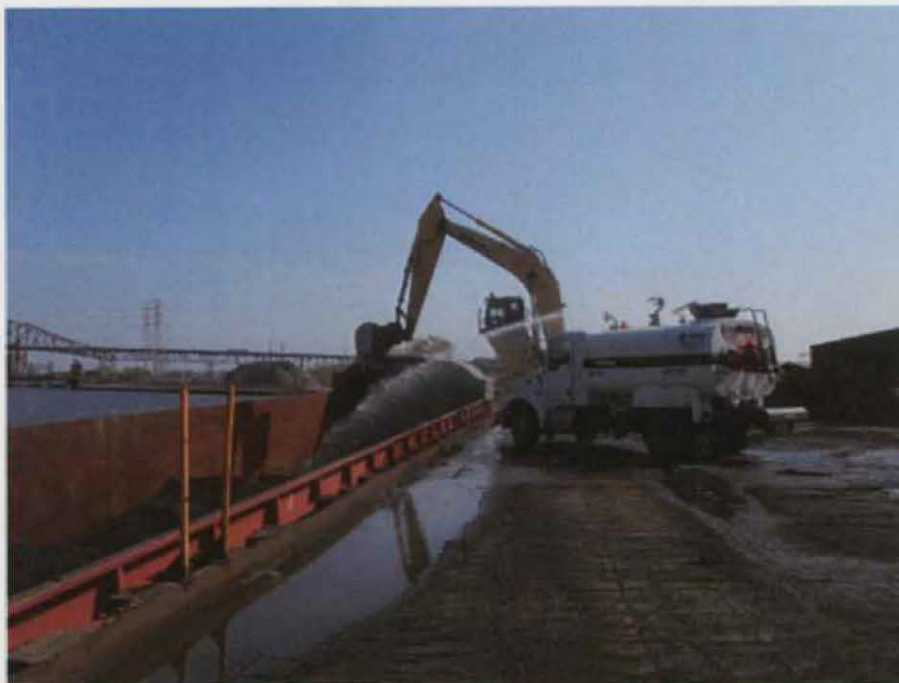
Photo 13. IMG_0373 at 9:14 am: Persistent watering during DRI unloading.
