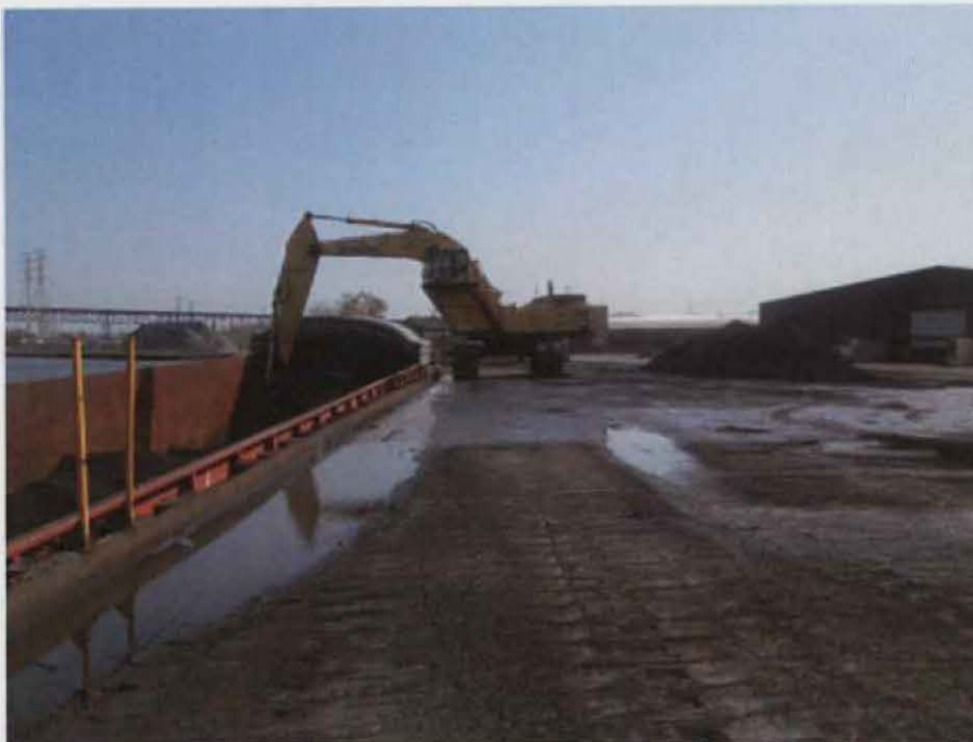
Photo 11. IMG_0371 at 9:09 am: DRI unloading.
