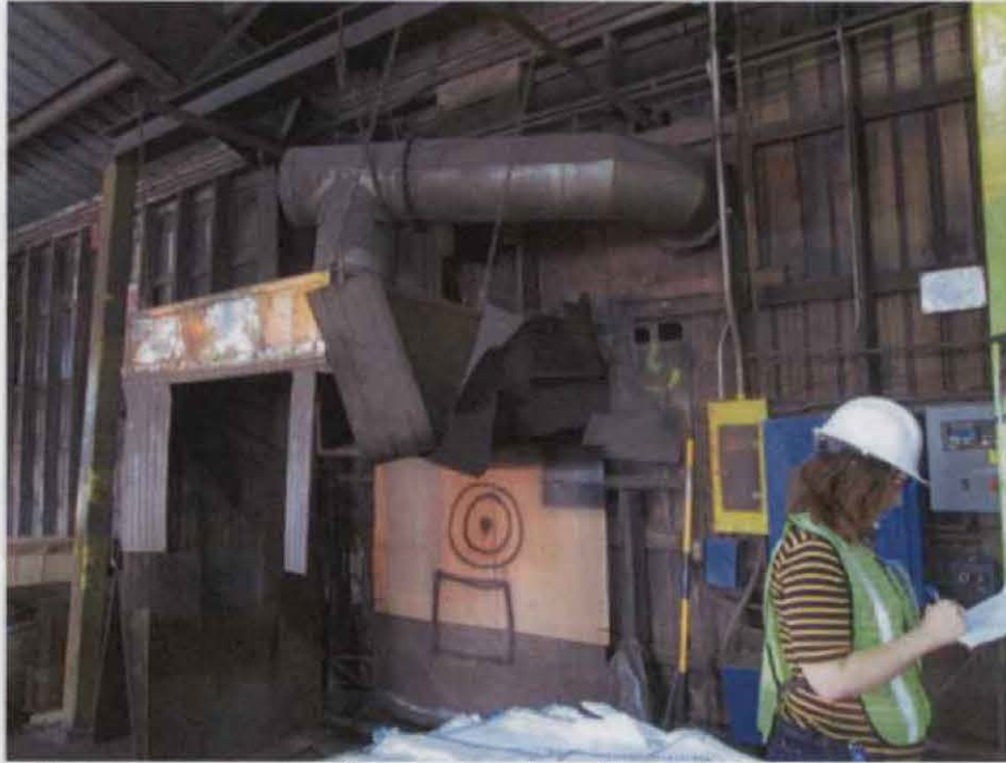
Photo 2. IMG_0360 at 8:11 am: SHB's Super Sack loading area.
