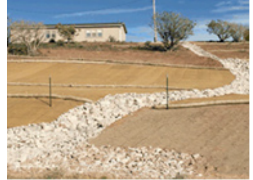
After: Slope stabilized
