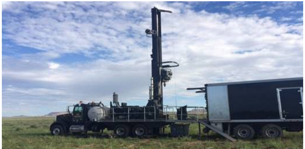
USEPA Conducting Soil and Groundwater Sampling Activities
