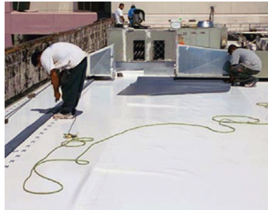
Figure 14: Installation of a Cool Single-Ply Membrane
