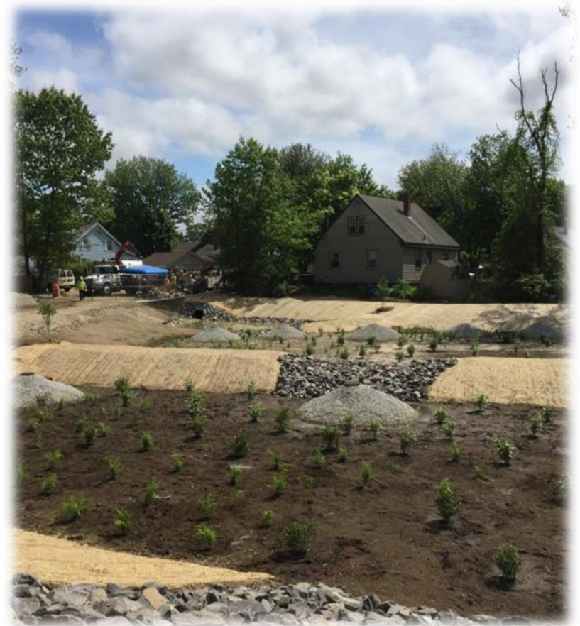
Bioretention & Subsurface Wetlands
