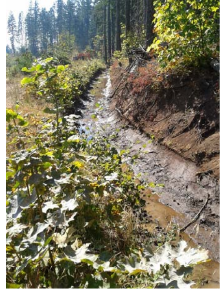
A canal prior to piping
