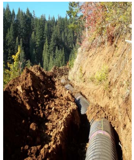
New pressurized irrigation pipe
