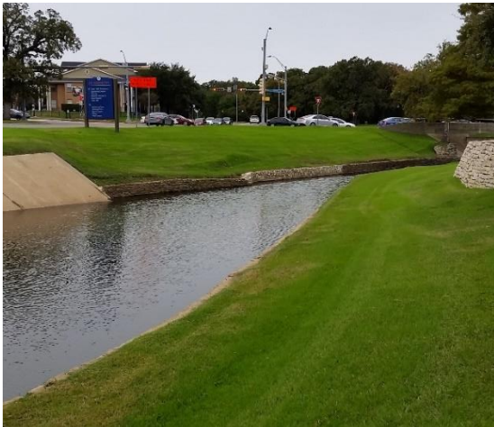
Figure 1 Showing partial concrete reinforcement of channel.
