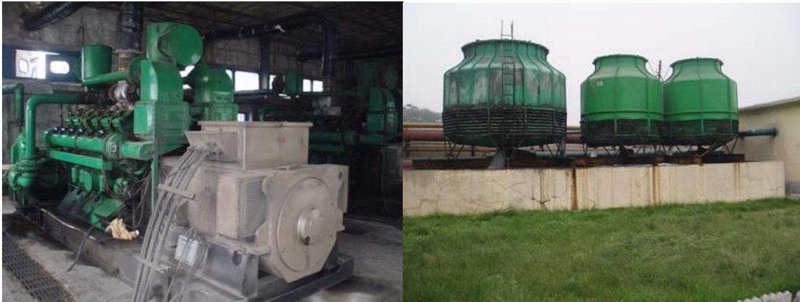
Exhibit 1-17: 500 kW Shengli Oil Company Generator Set and Waste Heat Recovery at Mine No. 6.
