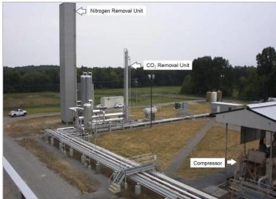
Exhibit 5-9 CO 2 Unit, Nitrogen Rejection Unit and Compressor (Adapted from Pena, 2007)
