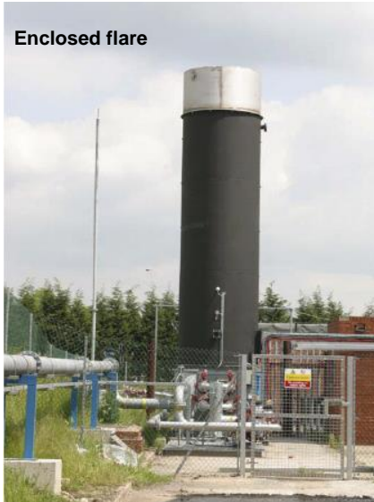
Exhibit 5-16: Enclosed and Open Flare Designs
