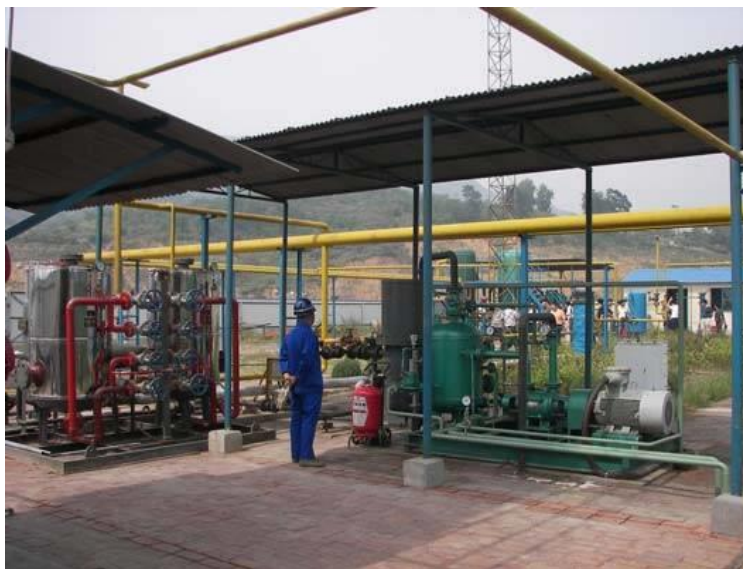
Exhibit 5-14: Yangquan CMM pilot project - compressor (right) and CMM purifier (left) (Yang, 2008)
