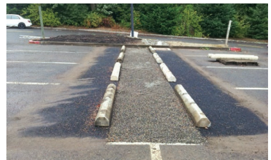
Figure 4. Paved tree well.
