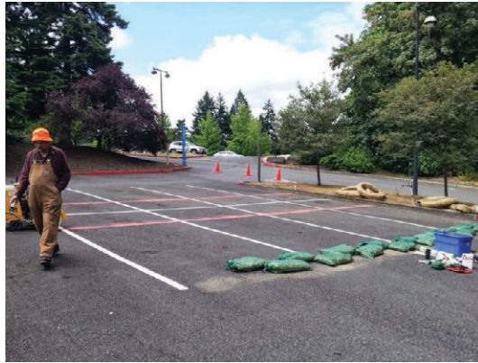
Figure 1. PCC parking lot, pre-construction.
