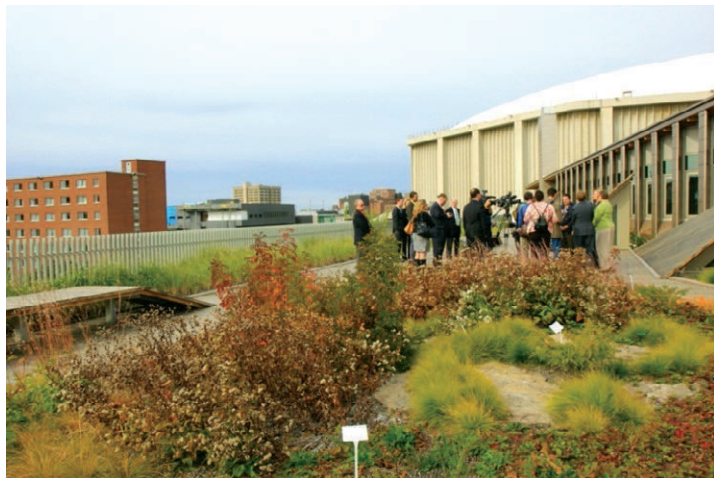
Green roof on top of Syracuse University's LEED Platinum certified Gateway Center. Photo Credit: Caitlin Eger, Syracuse Environmental Finance Center
