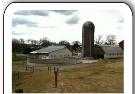
Pennsylvania uses CWSRF to support agricultural nonpoint source projects such as this manure storage facility. See page 11 .
