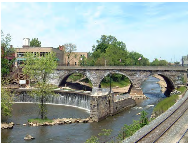
Figure 3. Project partners removed the lock and restored the river channel.
