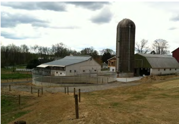
Figure 1. In the winter of 2011-2012, PENNVEST funds supported installation of this new concrete manure storage area and stabilized animal walkway at the Zook Farm in Lancaster County. For more project information see http://pacd.org/webfresh/wp-content/uploads/2012/05/Zook.pdf .
