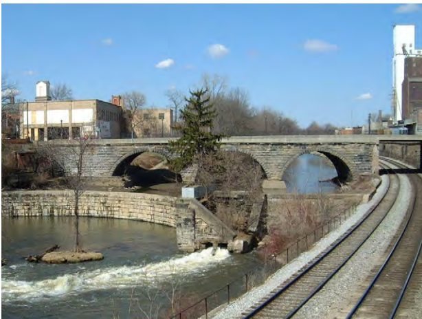
Figure 2. A lock on the right side of the stream channel created a pool behind the dam. The dammed water often became stagnant and contributed to poor water quality and aquatic habitat upstream.
