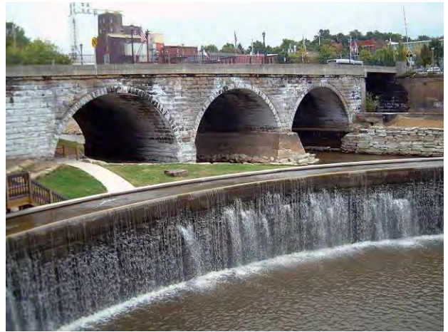
Figure 4. Partners replaced the old dam pool with a park. To preserve the look of the historically important dam structure and waterfall, project partners installed a pump to deliver water into a channel behind the dam that allows water to spill over into the river below.
