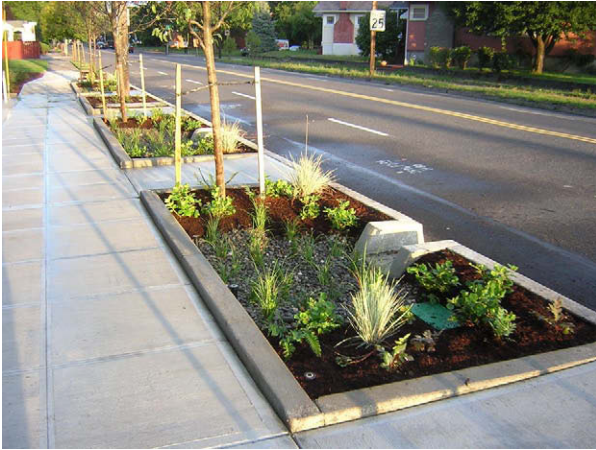
This stormwater planter captures and infiltrates runoff from the adjacent roadway.
