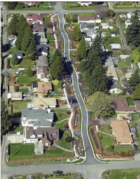
An aerial view of the SEA Streets project, immediately after construction.
