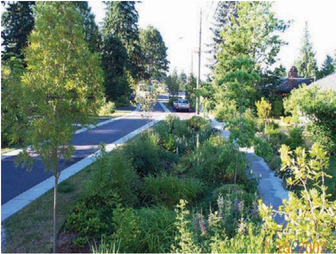
The Street Edge Alternatives—SEA Streets—project redesigned a typical residential block to include vegetated stormwater detention swales along a narrow, slightly curving street.
