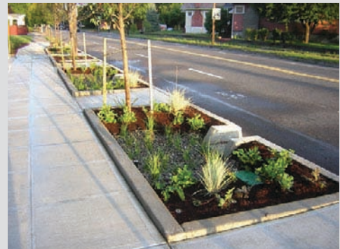
Portland, Oregon ( www.portlandonline.com/bes ) is a leader in the use of green infrastructure. These stormwater planters capture stormwater runoff and allow it to infiltrate. Any overflow backs up into the street and drains into existing storm drains.
