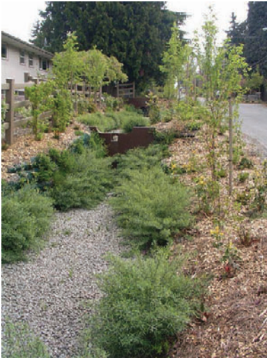
The 110th Cascade project replaced an existing ditch with a stair-stepped drainage system that slows water as it flows down a moderately steep slope.
