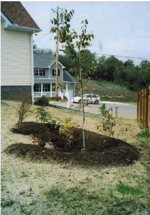
All downspouts from this BOB home at the Quiet Creek development lead into underground pipes that end with a pop-up valve into a rain garden.
