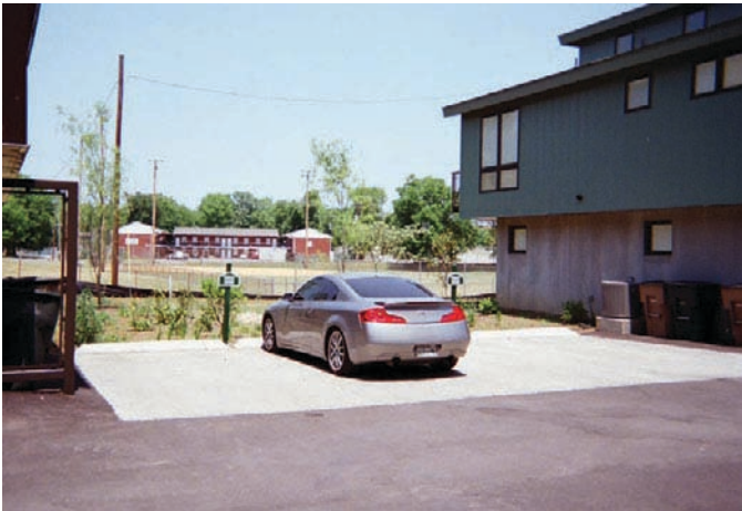
Morgan Park Place—an urban infill development—incorporates rain gardens and pervious parking areas to treat stormwater runoff from the roof and parking lot.
