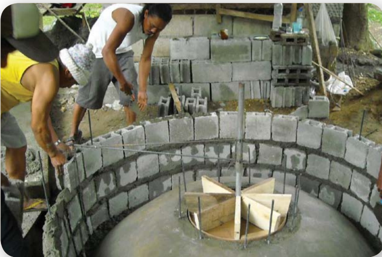
Stacked fixed dome digester construction at Nueva Vizcaya, Philippines.
