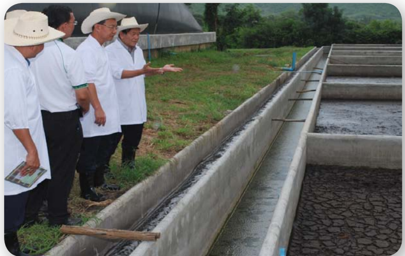
Sludge drying bed at Thailand's Kanchana Farm.
