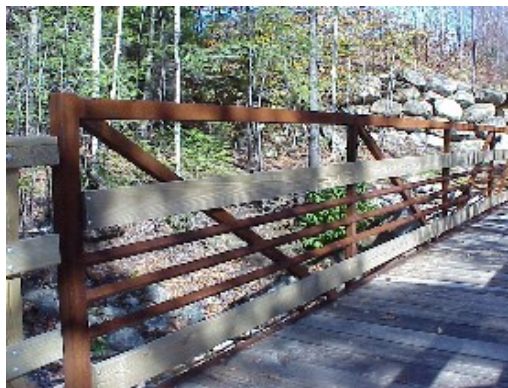
Figure 33: NH White Mountain Trail Bridge
