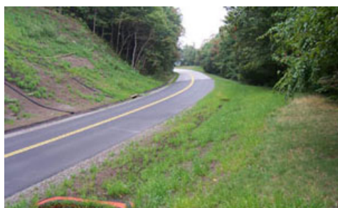
Figure 1919: Compost Blanket on Steep Slope on Federal Highway Helped Restore Slide and Re-establish Vegetation Restoration Despite Severe Drought
