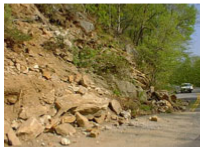
Figure 1919: Compost Blanket on Steep Slope on Federal Highway Helped Restore Slide and Re-establish Vegetation Restoration Despite Severe Drought
