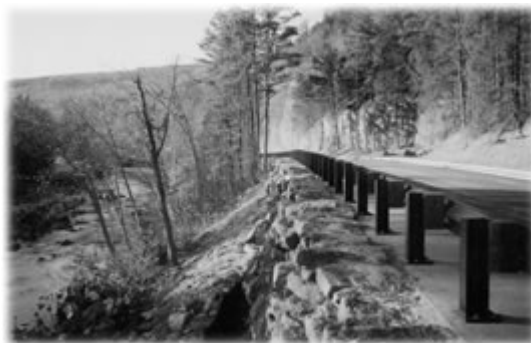
Figure 44: Arkansas SHDT Historic Bridge and Native Stone Retaining Wall
