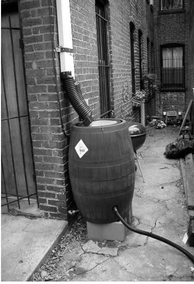
Rainbarrel attached to a rowhouse (DC WASA).
