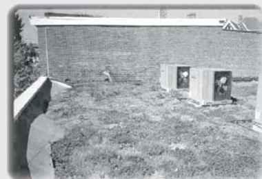
Photo: Roofscapes, Inc.
