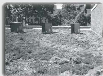
Photo: Roofscapes, Inc.
