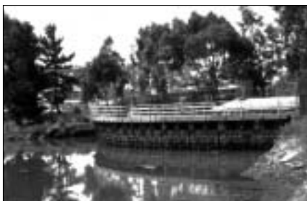
San Francisco's Islais Creek Transport/Storage Facility stores and conveys flow to the Southeast Plant. With a 600-foot overflow weir and 45 mgd storage capacity, this facility reduced combined sewer overflows from 40 to the allowable 10 per year.
