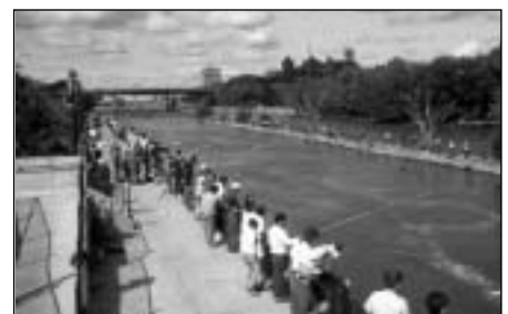
Fishing contest in Oswego, New York, a CSO community that has implemented the NMC and structural controls, including a swirl concentrator and disinfection system.
