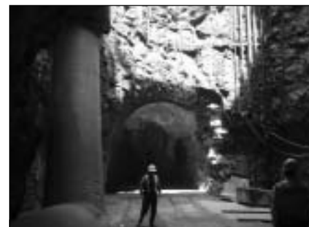
Richmond, VA has been implementing CSO controls since the early 1980s. The storage tunnel at the Falls of the James River, shown, is part of the second phase of a plan that included increased wet weather storage and treatment capacity.
