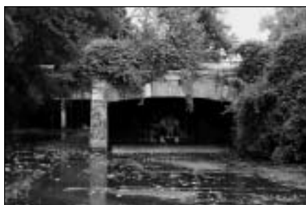
CSO outfall to Piney Branch, Washington, D.C.
