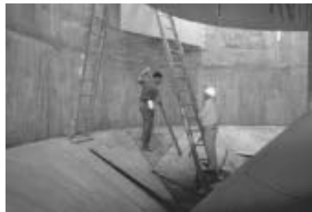
Vortex separation facility under construction. Courtesy of Columbus Water Works.
