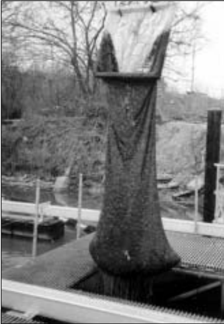
Floatables control is accomplished through pollution prevention activities such as street cleaning and public education, and through physical controls, such as this netting system serving the Cleveland, Ohio area.
