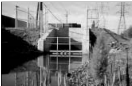
Floatables control facility in North Bergen, New Jersey.
