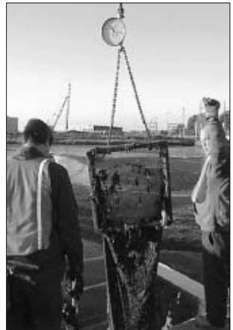
New Jersey provides CSO communities with planning and design grants for solids and floatables control measures, such as nets like the system used in North Bergen.
