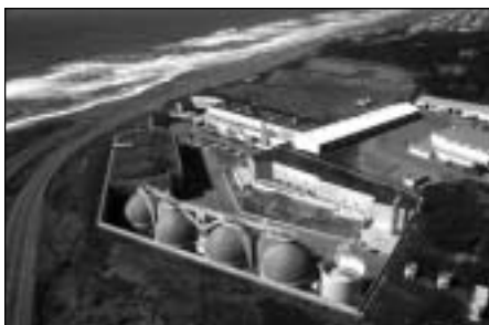
San Francisco's CSO Oceanside Water Pollution Control Plant treats an average of 17 mgd during dry weather and has 65 mgd peak flow capacity. During wet weather, excess flow is stored in structures that remove sediment and floatables before the flows are transported to the plant for treatment.
