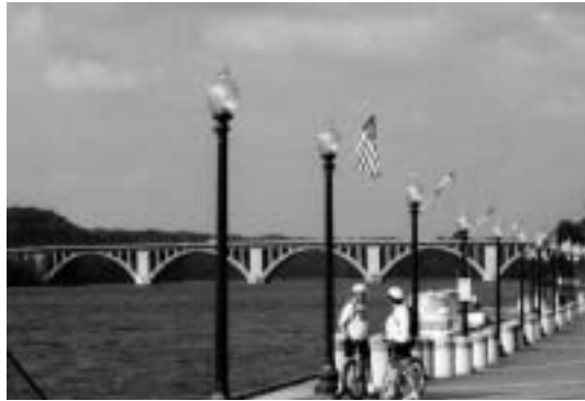
Photo: Potomac River in Georgetown, Washington, D.C. Courtesy of Greeley & Hansen Engineers, Inc.
