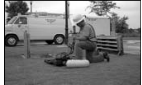
Most states require CSO BMPs in permits. Of the NMC, the first six measures are the most widely implemented.
