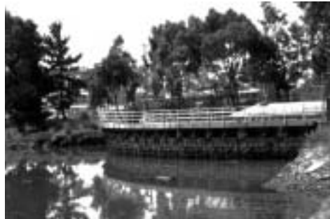
Photo: Islais Creek CSO Wet Weather Treatment and Storage Facility Courtesy San Francisco PUC
