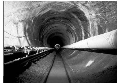
EPA and the State of Georgia consolidated enforcement efforts to resolve CSO and other water quality violations in Atlanta. This new sewer tunnel is part of the city's remedial action plan.
