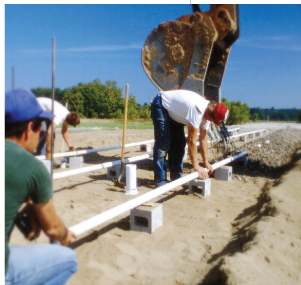
Mound system under construction (photo courtesy of Ayres Associates)
