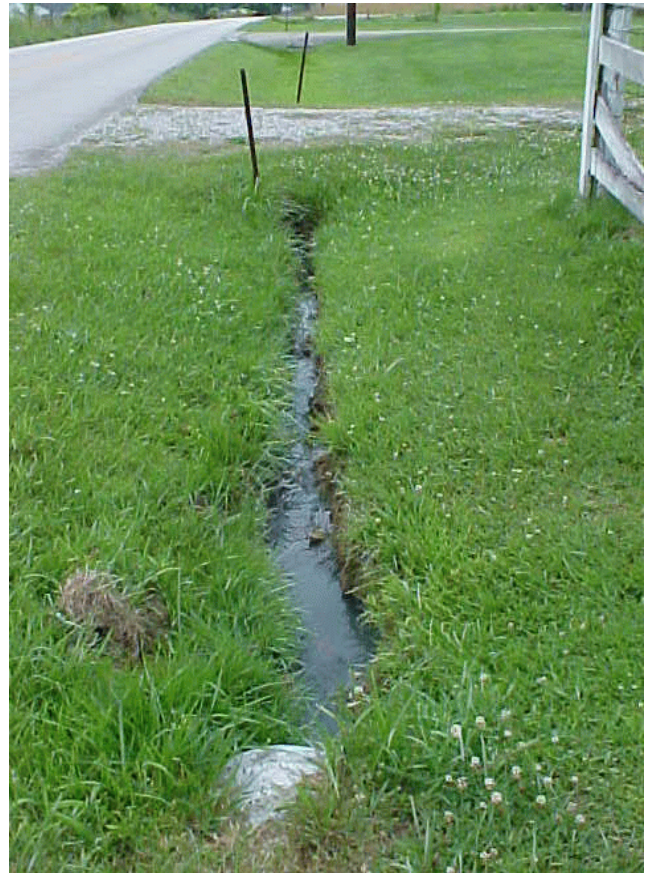
Straight Pipe Drainage: Preston, KY
