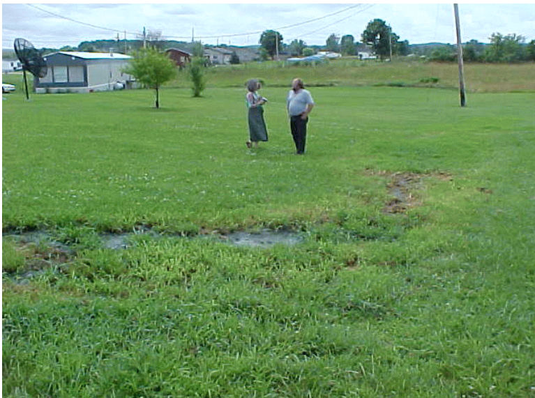
Failed Septic System: Preston, KY
