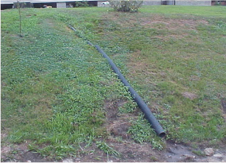
Straight Pipe: Martin County, KY
