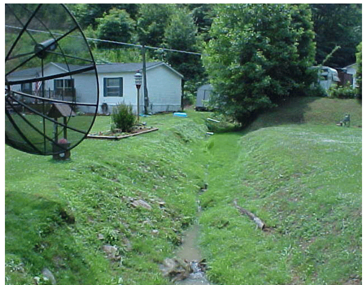
Straight Pipe Drainage: Kermit, West Virginia
