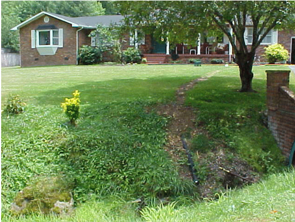
Straight Pipe: Martin County, KY
