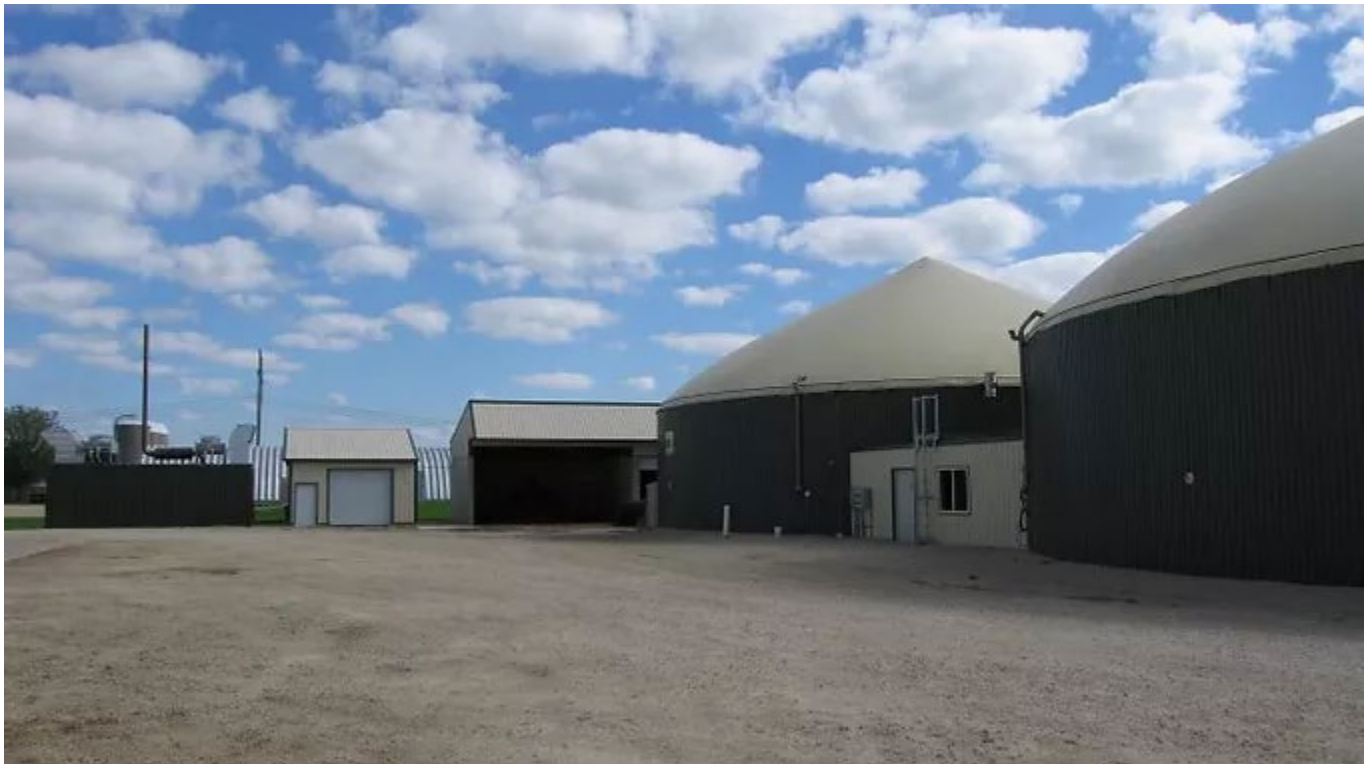
Complete mix anaerobic digesters at Vir-Clar Farms. Photo Credit: Vir-Clar Farms
