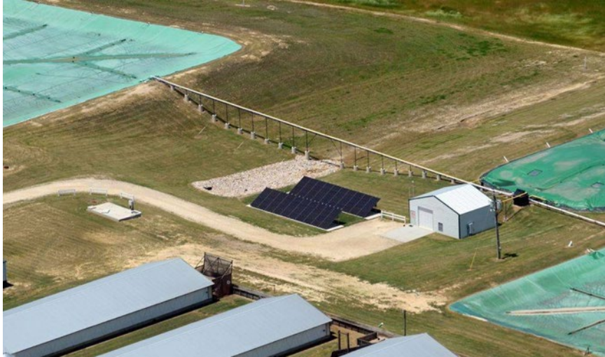
Finishing barns, waste mix tank, solar panels, generator shed, covered lagoon digester, and two covered effluent lagoons.
