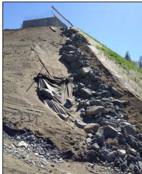
Figure 16. Development on steep slopes and poor erosion control methods can cause erosion and increase the quantity of stormwater runoff. Steep slope development regulations can help prevent some of these impacts. Credit: Vermont Stormwater Program.
