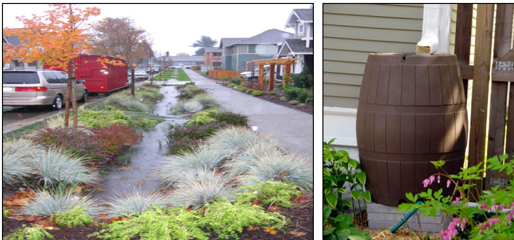
Figure 15. Green infrastructure techniques such as rain gardens (left) and rain barrels (right) retain stormwater runoff on site and reduce peak flooding. Credit: Clarion Associates.
