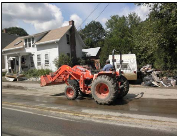
Figure 12. There was extensive cleanup work in Moretown, Vermont after Tropical Storm Irene. Credit: Stephen Magill, Vermont Department of Environmental Conservation.
